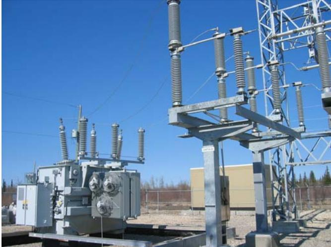
The spare transformer connected to the transmission system (“on potential”)
