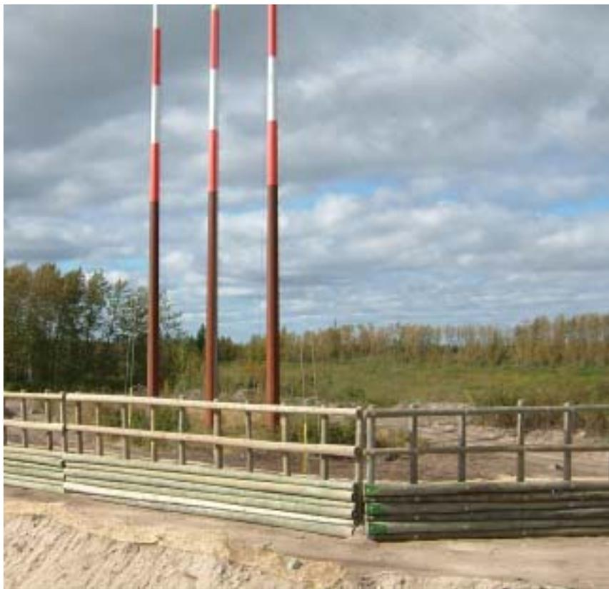
*Berms have been built at major river crossings to protect the transmission line from damage at breakup*
