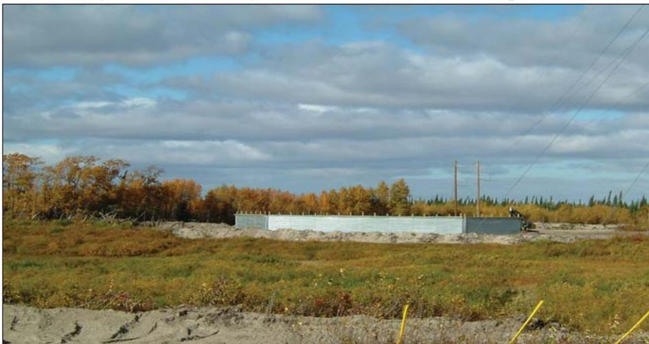
The new berm built to protect Structure 909 from ice-jamming during spring break-up.
