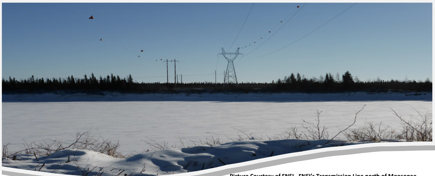
Picture Courtesy of FNEI– FNEI's Transmission Line north of Moosonee.
