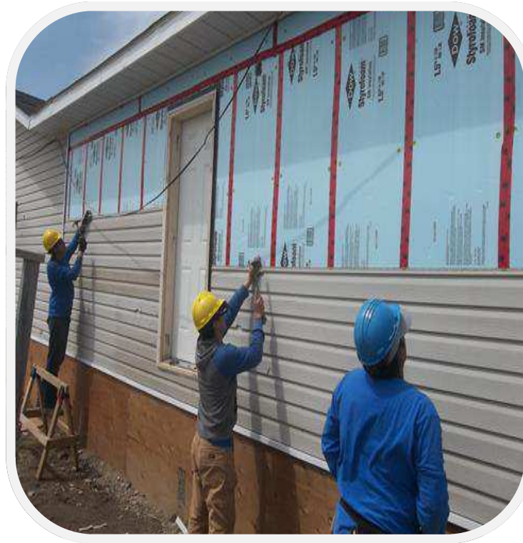
Men at work installing siding over new layer of wall insulation.
