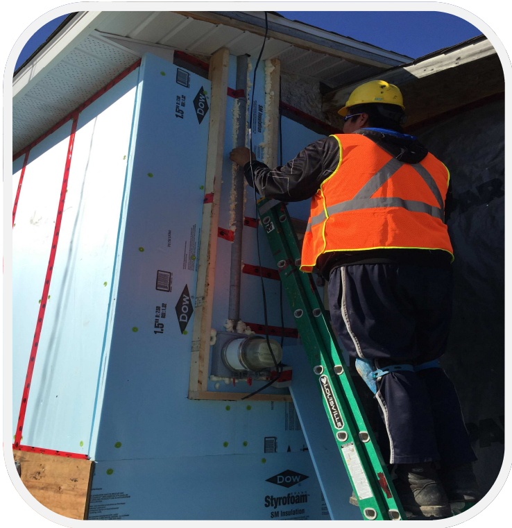
A Community worker for the Conservation on the Coast program installing wall insulation and air sealing a house.
