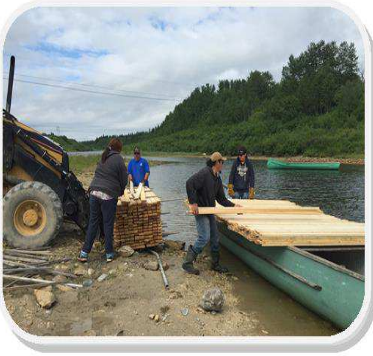
Wood Strapping made in Fort Albany is on its way to Kashechewan for use behind the siding.
