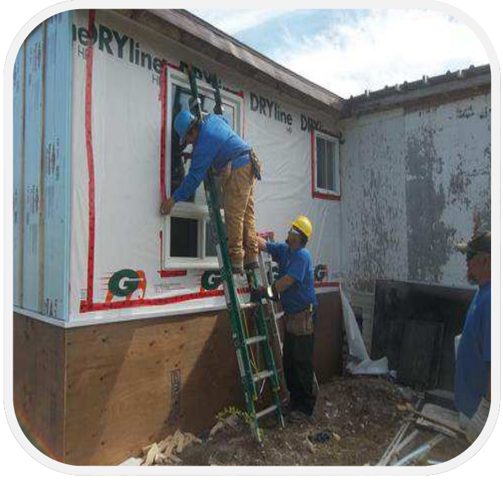
Men at work installing the air barrier to stop cold drafts.
