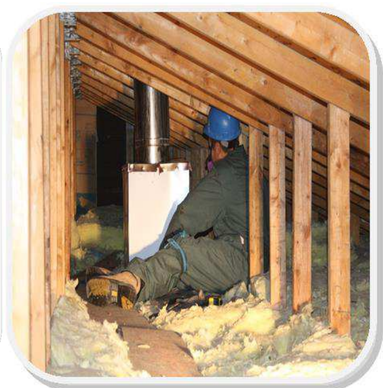
Here you see a Community worker making a baffle around a chimney before adding more insulation to the attic.
