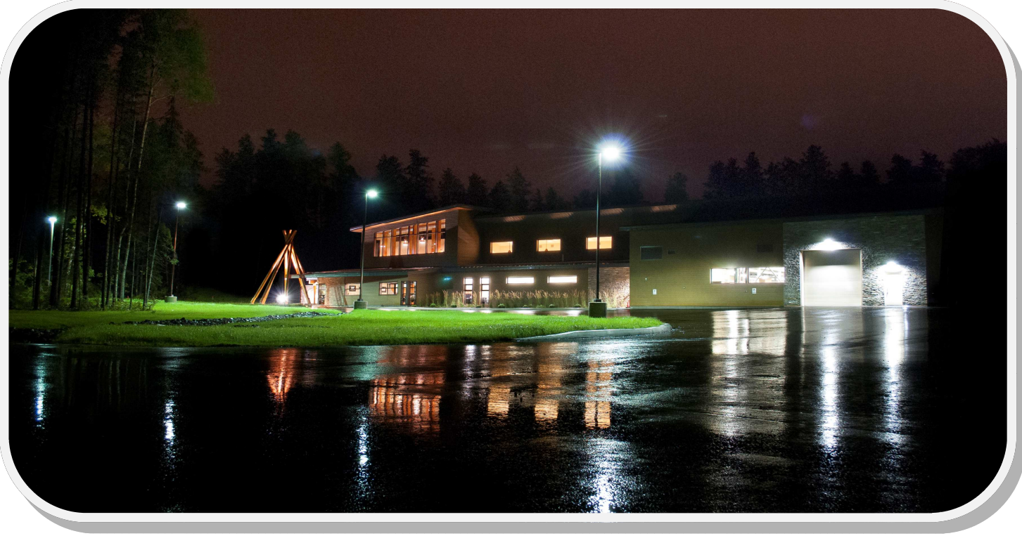
Above: Night picture taken of FNEI’s new office building. This is the culmination of efforts by FNEI to address the increasing need for more space, and with increasing staff requirements in the technical department, etc.
