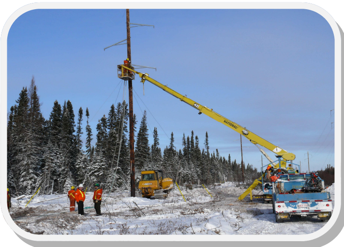
Crew hard at work stringing up transmission lines.
