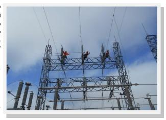
PowerTel crew (above) installing new disconnect switch for bus section.  $< D \le U^T \quad b \le C P \quad b \quad A \le C P \cap C P \quad A \le C P$
