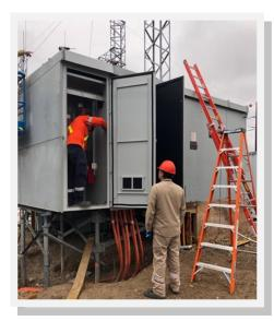
New cell added to the existing switchgear, to improve Attawapiskat distribution system configuration and increase reliability. (*last one on the left*)
