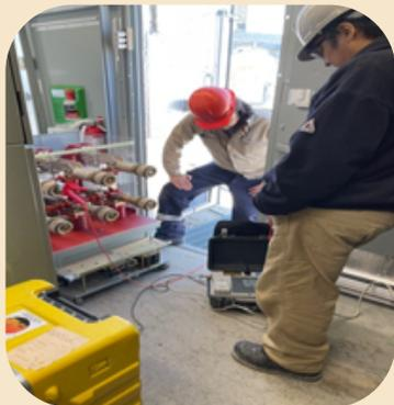
Ryley and Bobby testing insulation values on a medium voltage breaker
