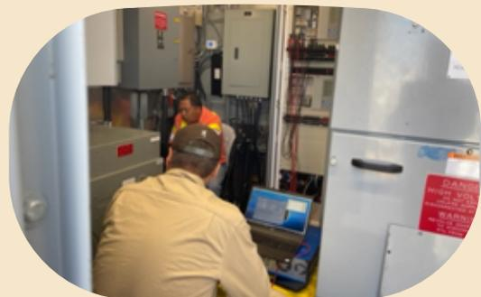
Bobby and Steven Xue, a FNEI contractor, performing a function test for a line protection relay for K5A, the line from Kashechewan to Attawapiskat
