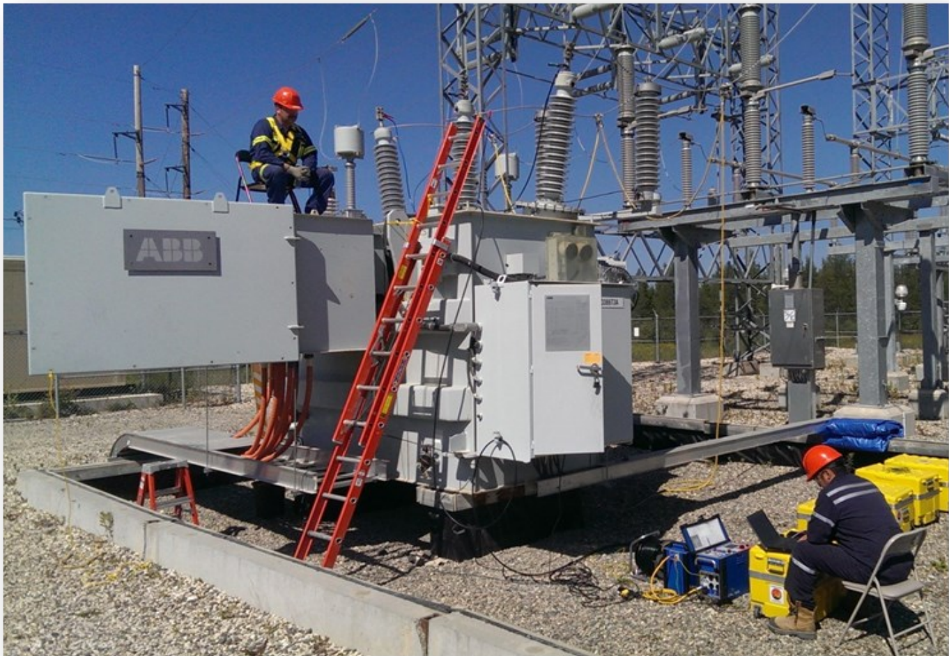
Above: Robert Chookomoolin and Stephen Firlotte testing transformer, summer 2014.
