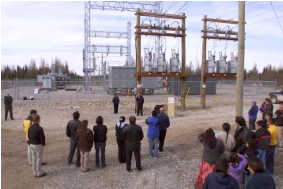
The crowd gathers at the Fort Albany substation for the ribbon cutting ceremony.
