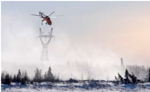
A helicopter installs the top section of the high voltage support.
